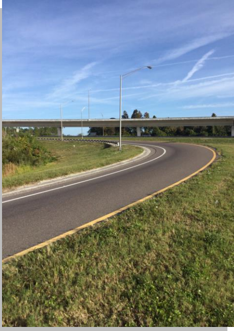
Figure 1: Selmon Expressway EB Exit Ramp to 78 th St
