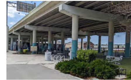
Park Use Under Expressway
