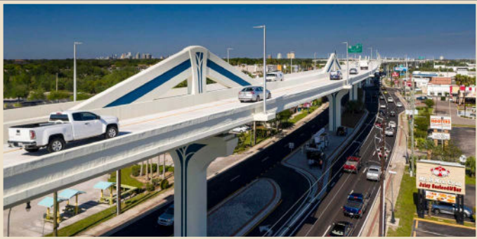
Existing Bridge Conditions
