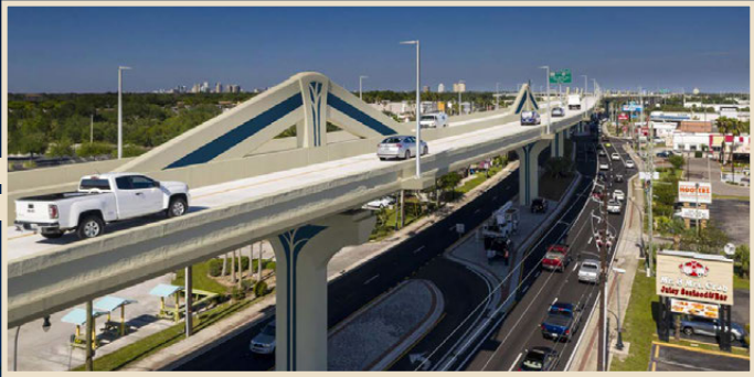
Proposed Bridge Aesthetic Features
